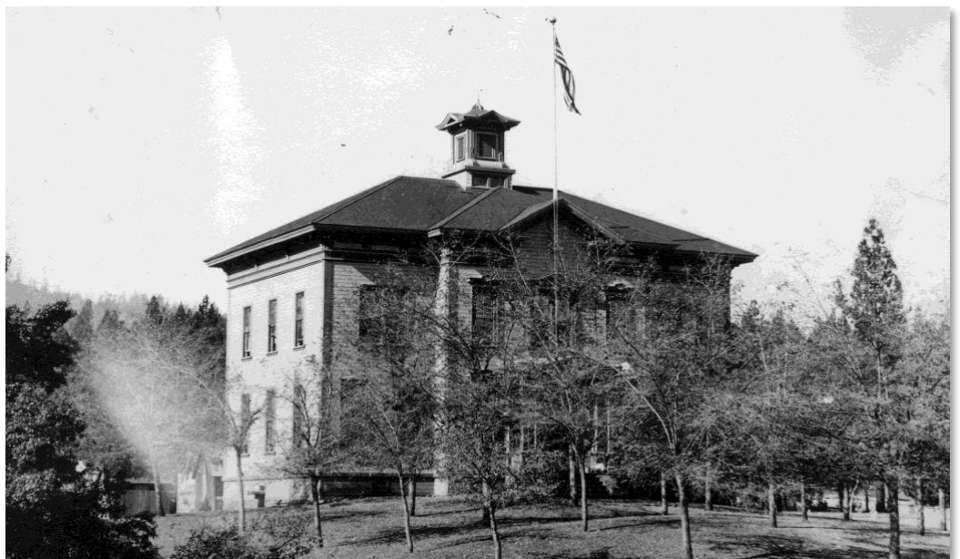
Weaverville School House, 1903
