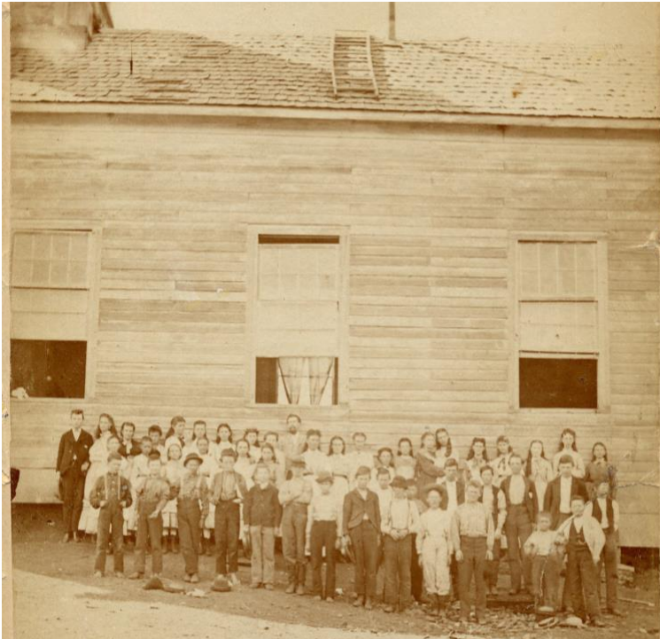
Weaverville School House 1874
